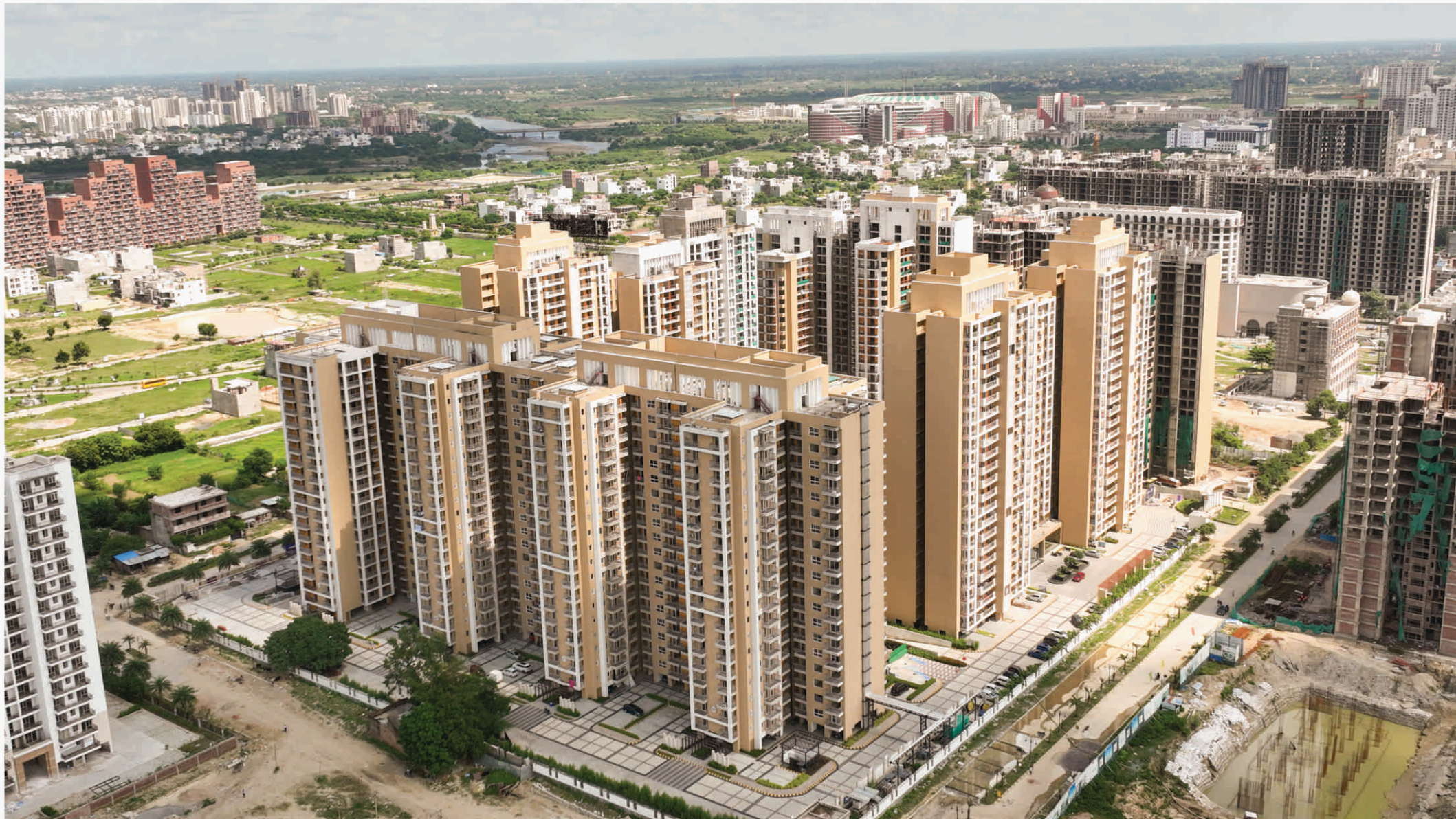
FINISHING WORK IN PROGRESS
